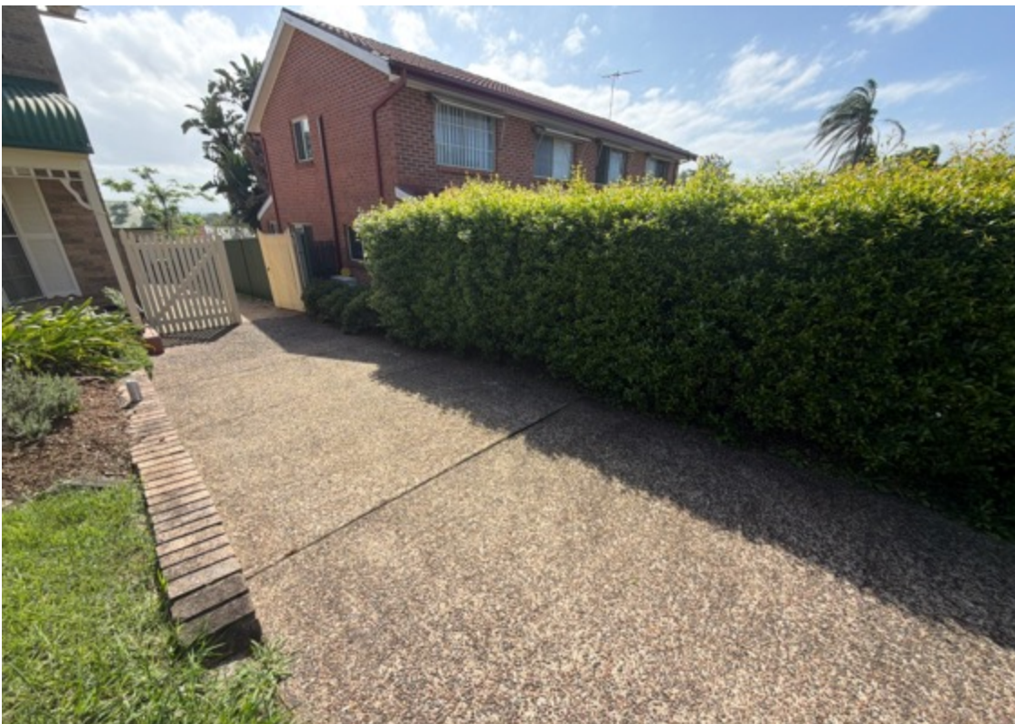
Isolated sections of exterior concrete displays typical shrinkage cracks and undulations - consistent with age.
