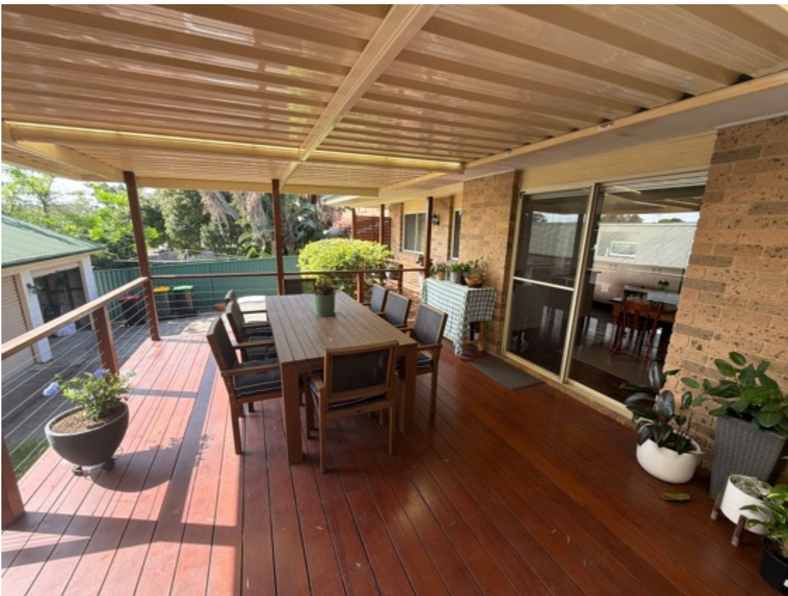
The rear pergola checked is structurally sound.
