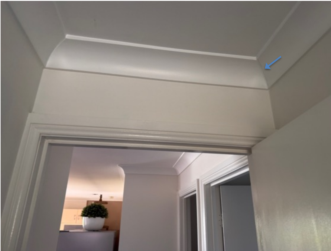
Isolated sections of plasterboard and cornices are cracking (common toilet example above.)
