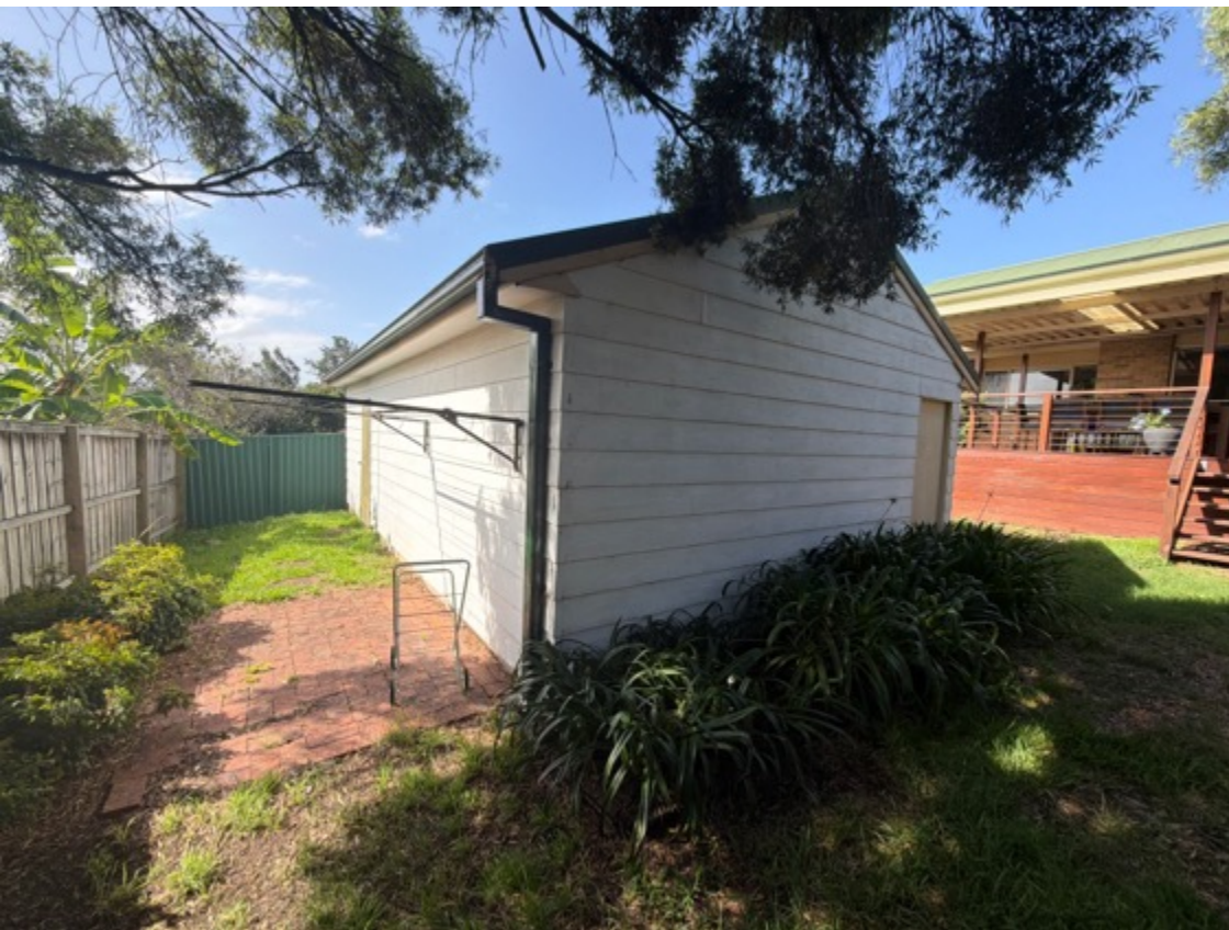
Surfaces are moderately paint blemished and timber is weathered, consistent with age.
