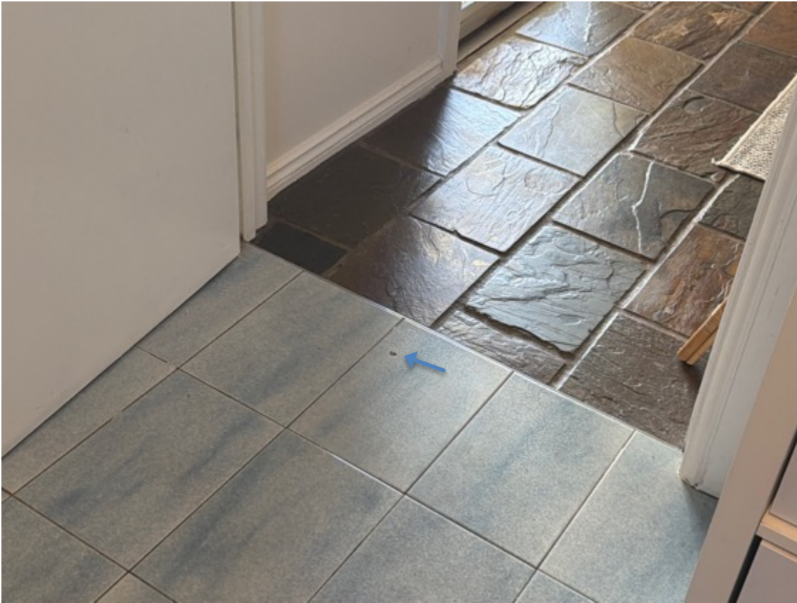
Isolated sections of tiles are chipped, consistent with age.
