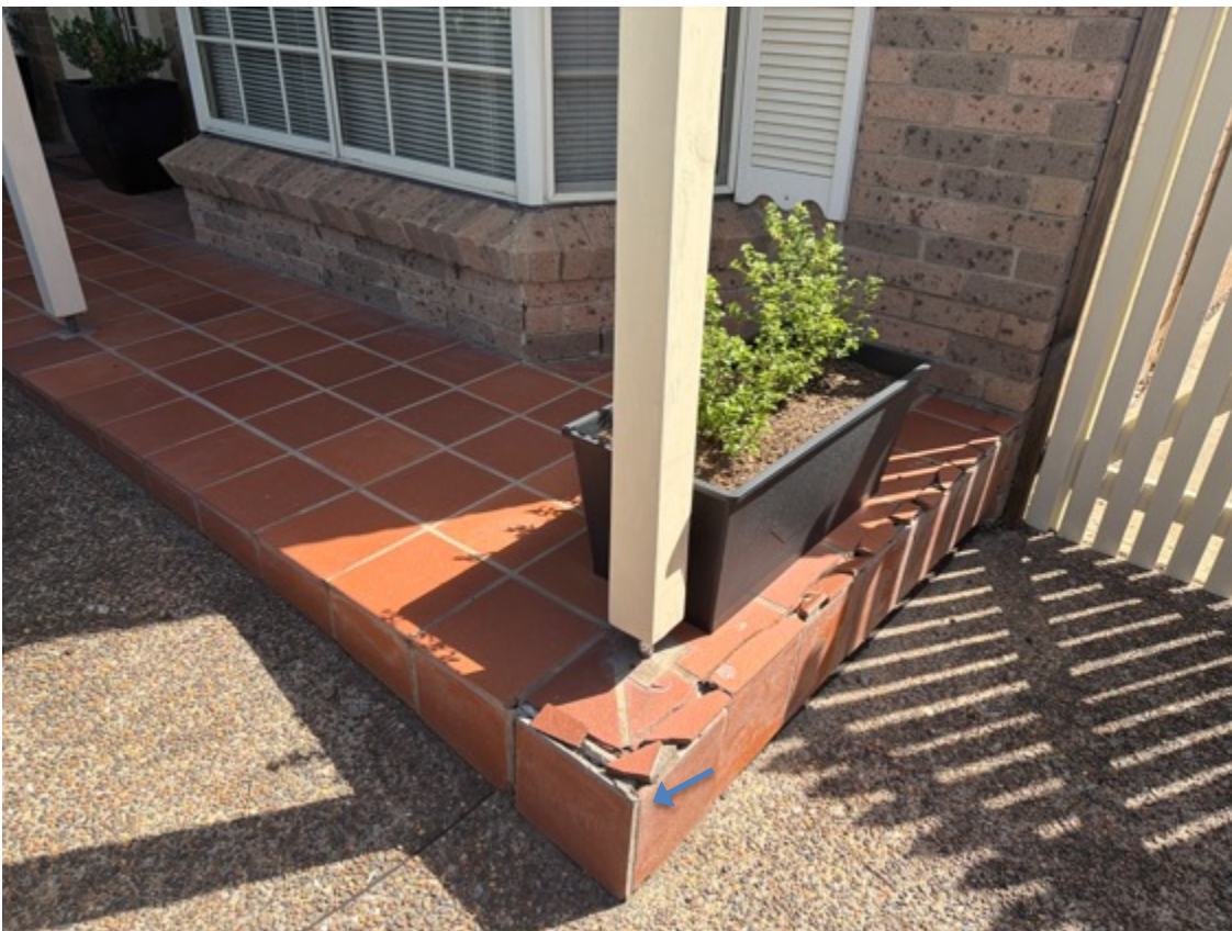
Isolated sections of external tiles are cracked, consistent with age.
