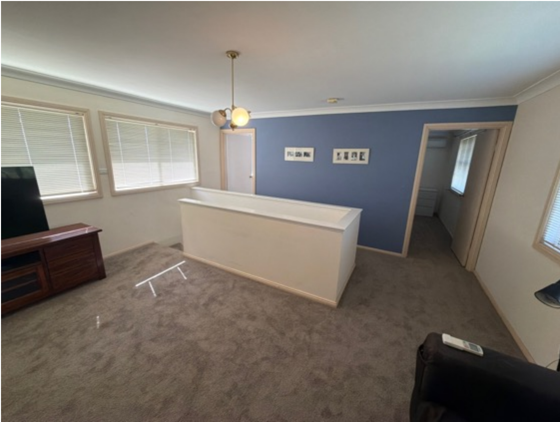
Interior railings checked are structurally sound.
